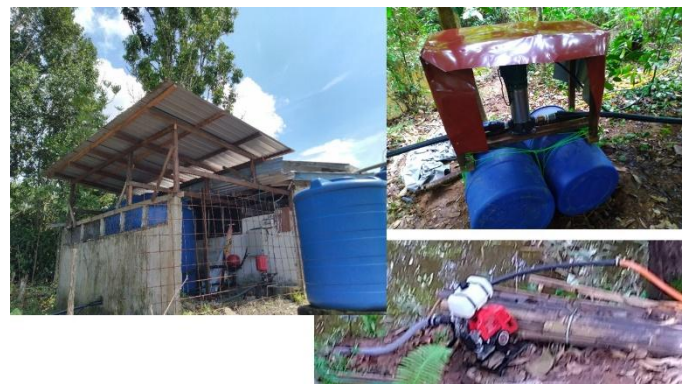
Fig. 9. Left is the pump house; right top is the 4 HP pump near the river and bottom right is the combustion engine pump. The two red pressure booster tanks are for the 1 HP and 4 HP tanks, the specification of which are in Table 3.
