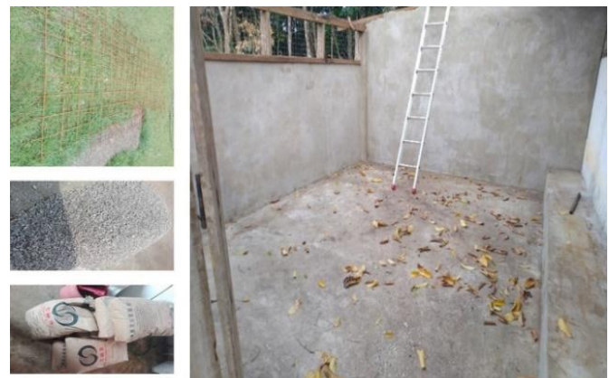
Fig. 3. The BRC, gravel, cement and sand and the reinforced floor to place the 9000L holding tank
