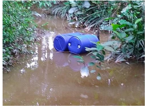
Fig. 11. The incoming 1½" HDPE incoming pipe is tied below the two blue drums float which are fastened together with truck ratchet ropes
