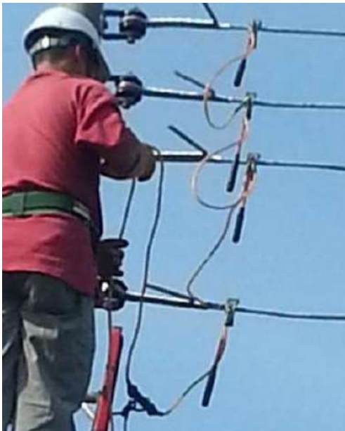
Fig. 19. This method can be used to get 3 \Phi power from the LV side of substations
