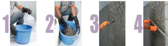
Fill a clean pot with potable water measuring 18% (+/- 5%) the weight of Sandfree Plaster (1 kg Sandfree Plaster : 0.18 litres water).
