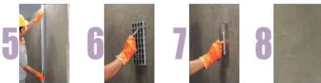
After initial setting apply aluminium scrapping patty to achieve true level and create a rough texture for subsequent coat.
