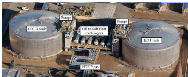
Fig. 2 Storage tank for Solar Two power plant
